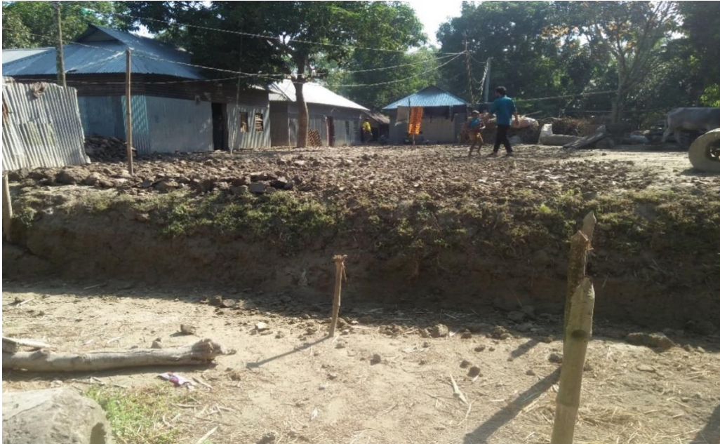
Plinth raise through a community approach at Dhontotla, Belgacha, Islampur in Jamalpur
