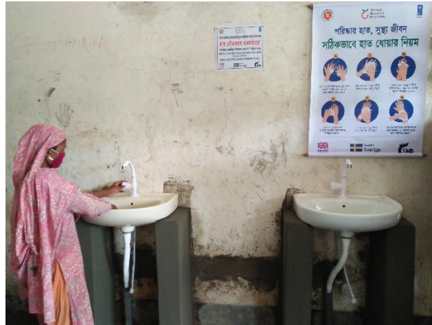
Use of hand washing point to protect against COVID-19 at Belgachha Flood Shelter center
